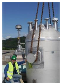
Destillationskolonne Ø 2400 x 22000 mm
