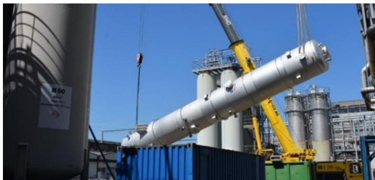
Destillationskolonne Ø 2400 x 22000 mm
